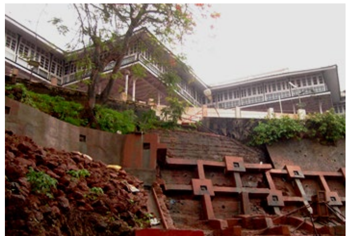
Real time geotechnical monitoring from a historical monument on a hill.
