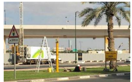
Geodetic data from existing bridge monitoring near deep excavation
