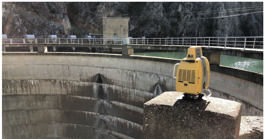
Online monitoring of existing dams, as well as dams during construction
